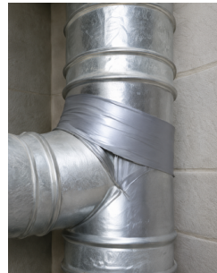
DUCT SEALING / HVAC REPAIR
